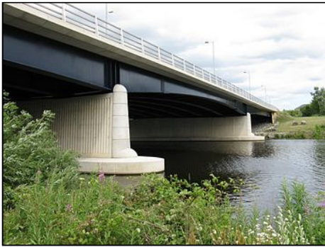
Photos 15, 16, and 17: High Quality Concrete finishes on bridge piers
