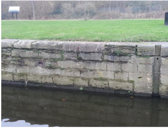
Photo 7: Typical material along Knostrop Cut
