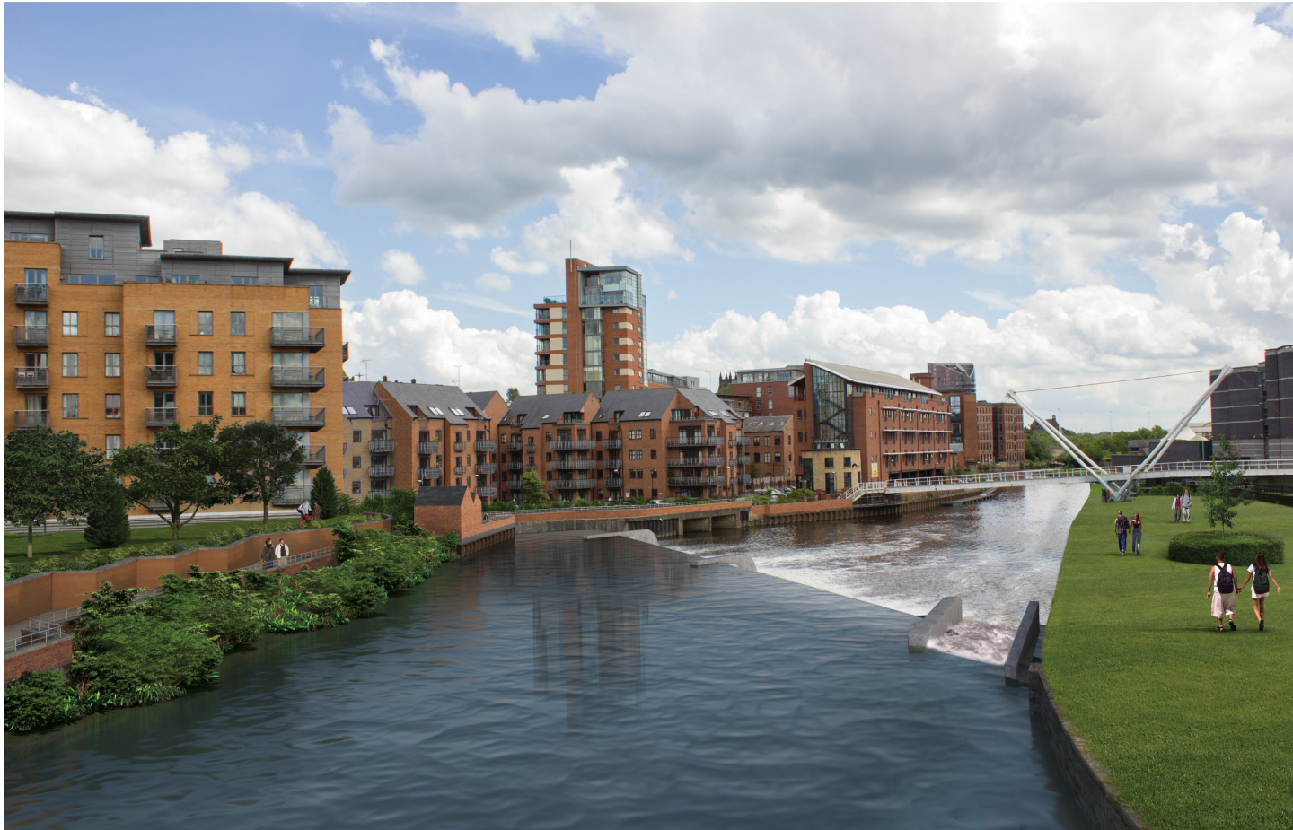
Figure 6: Upstream visual representations of Concrete finishes
